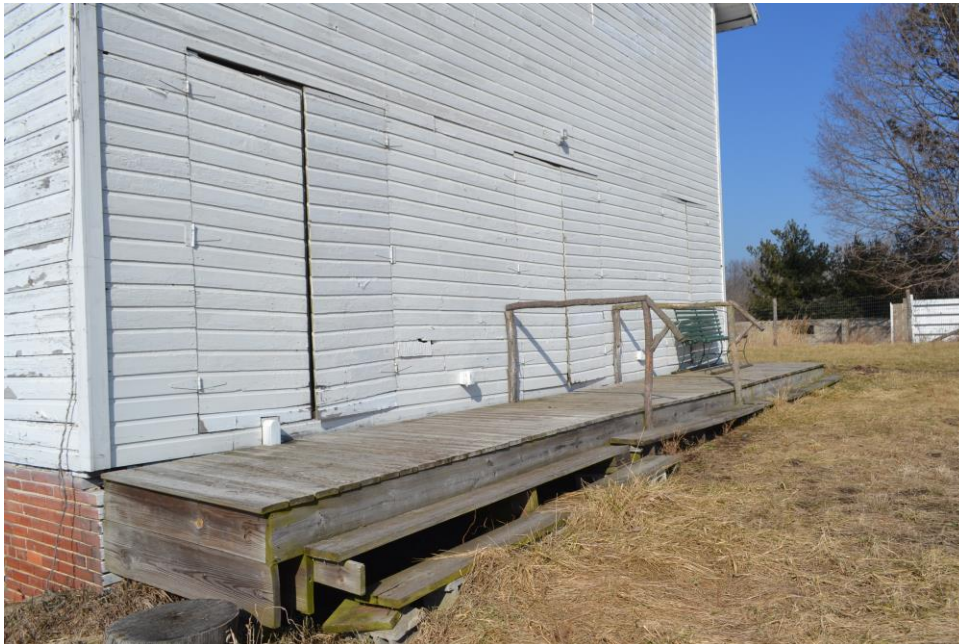
8. Recommended removal of deck for basement masonry wall repair. A new deck may be installed after repair.
