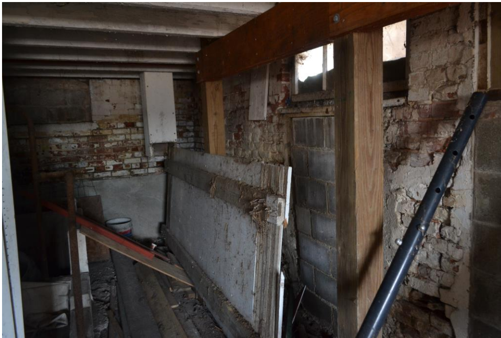
25-26. East basement wall showing masonry deterioration from moisture penetration. This area also appears to have been at least partially exposed with grade raised on the exterior. This end also includes new column and beam construction for reinforcement of main level floor.
