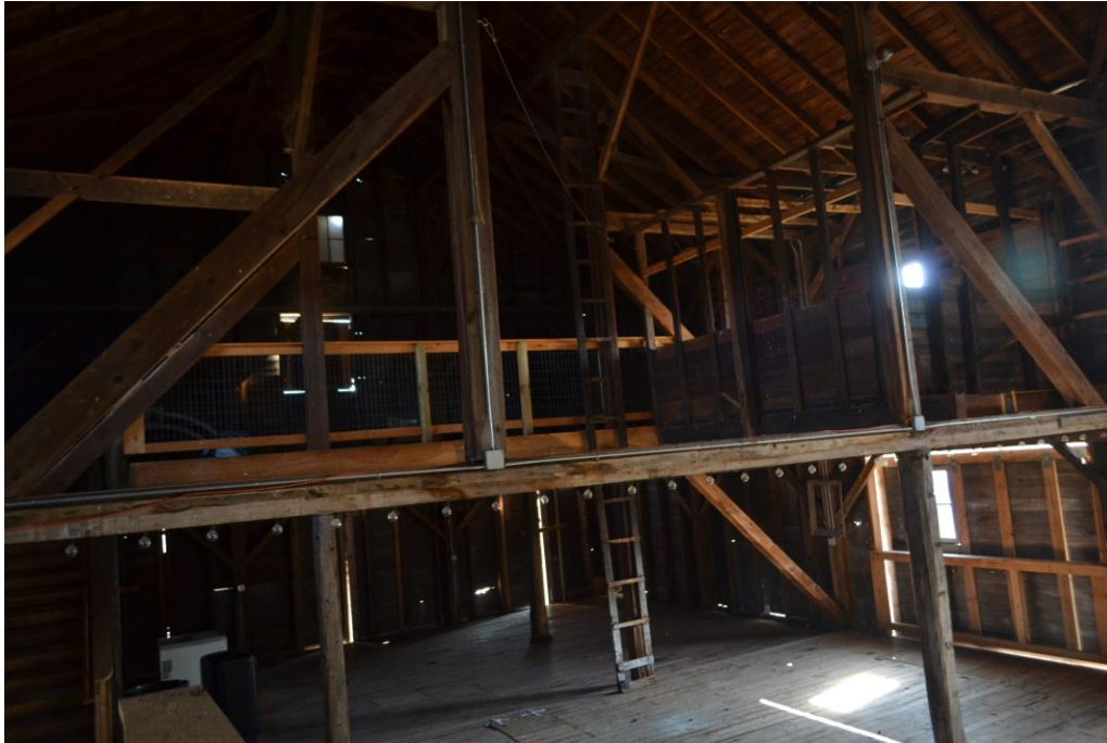
17. Looking east (top) and 18. northeast in east loft (bottom). Note missing structural post in top photo and existing, but covered gable window in bottom photo.
