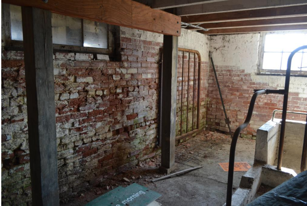
25-26. East basement wall showing masonry deterioration from moisture penetration. This area also appears to have been at least partially exposed with grade raised on the exterior. This end also includes new column and beam construction for reinforcement of main level floor.
