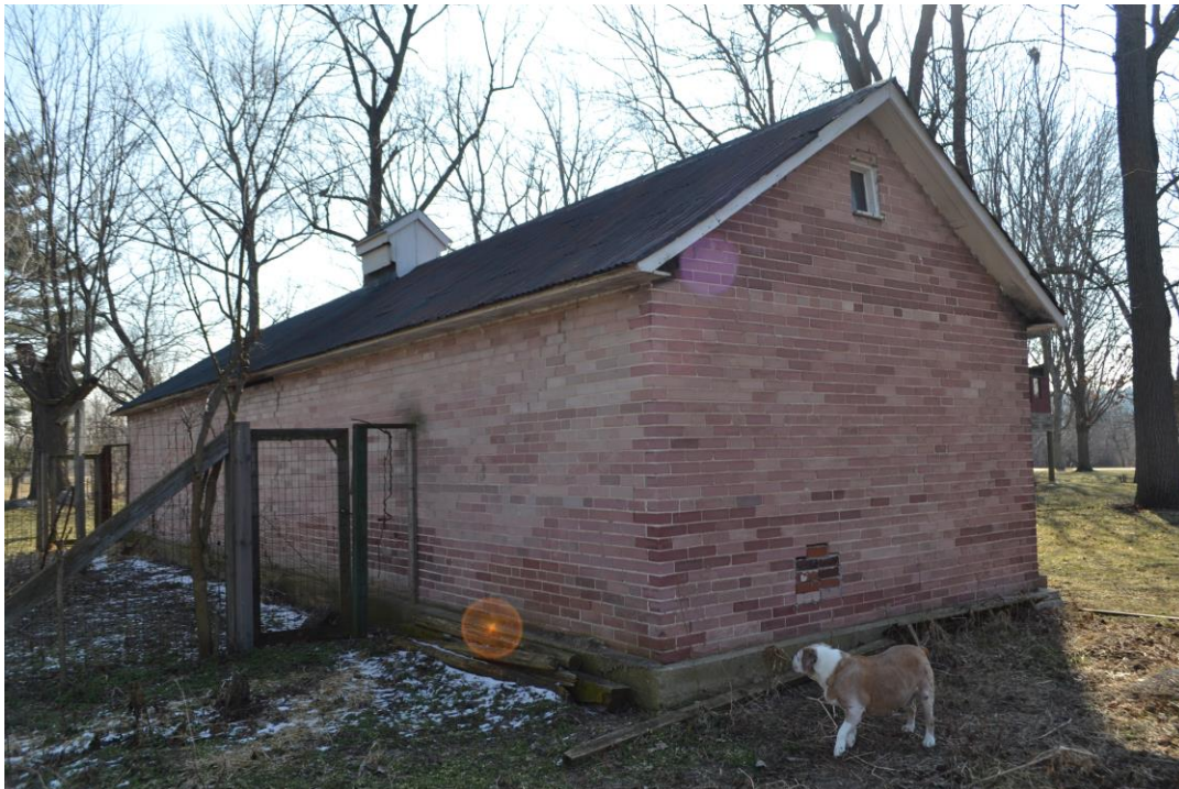
35-36. Chicken Coop. Above note inadequate mortar parging on front wall and settlement over modern metal entry door. Below note obvious settlement in mortar joints on back (north) wall.
