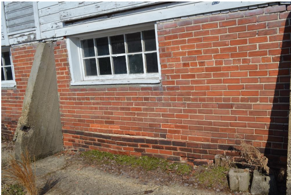
6. One of the most significant failures is a separation of face brick from the lower wall. It is unclear why the separation is occurring, but this can be removed and re-laid.
