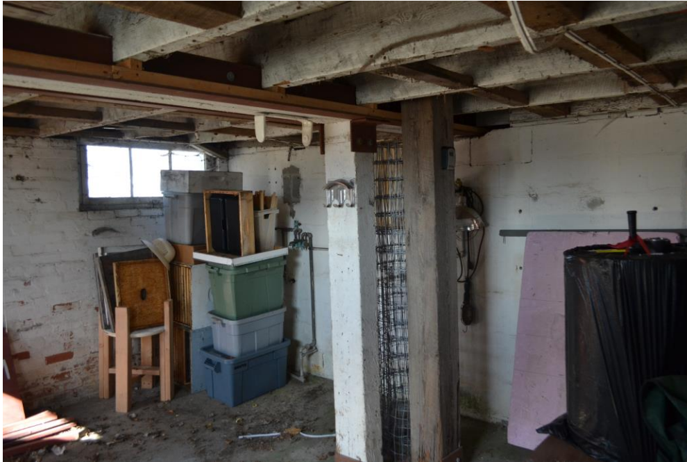
33-34. Dairy office in southwest corner features modest renovations and reinforcement, including masonry wall reinforcement along base of south basement masonry wall. Concrete buttresses were installed outside of the south wall sometime as an early reinforcement.
