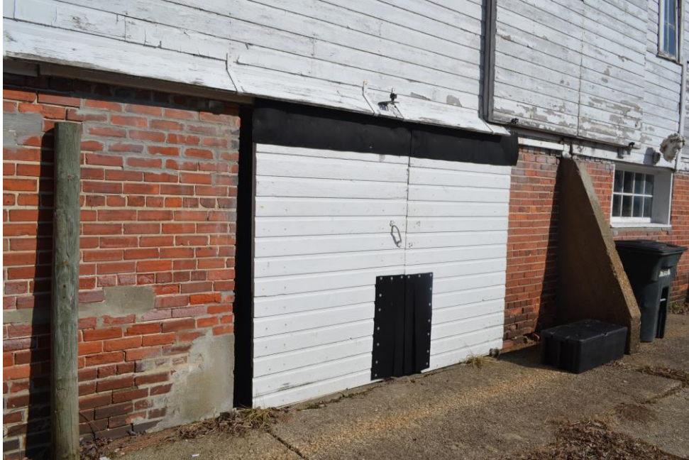
5. Inadequate masonry mortar repair that occurred in previous years should be addressed
