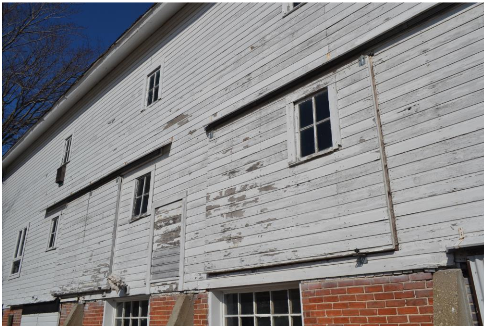
12. Aside from perimeter drainage issues, the exterior is in fairly good condition. Wood siding is in good condition with limited need for repair/replacement. Paint failure will require future scheduling of scrape/prime/paint.
