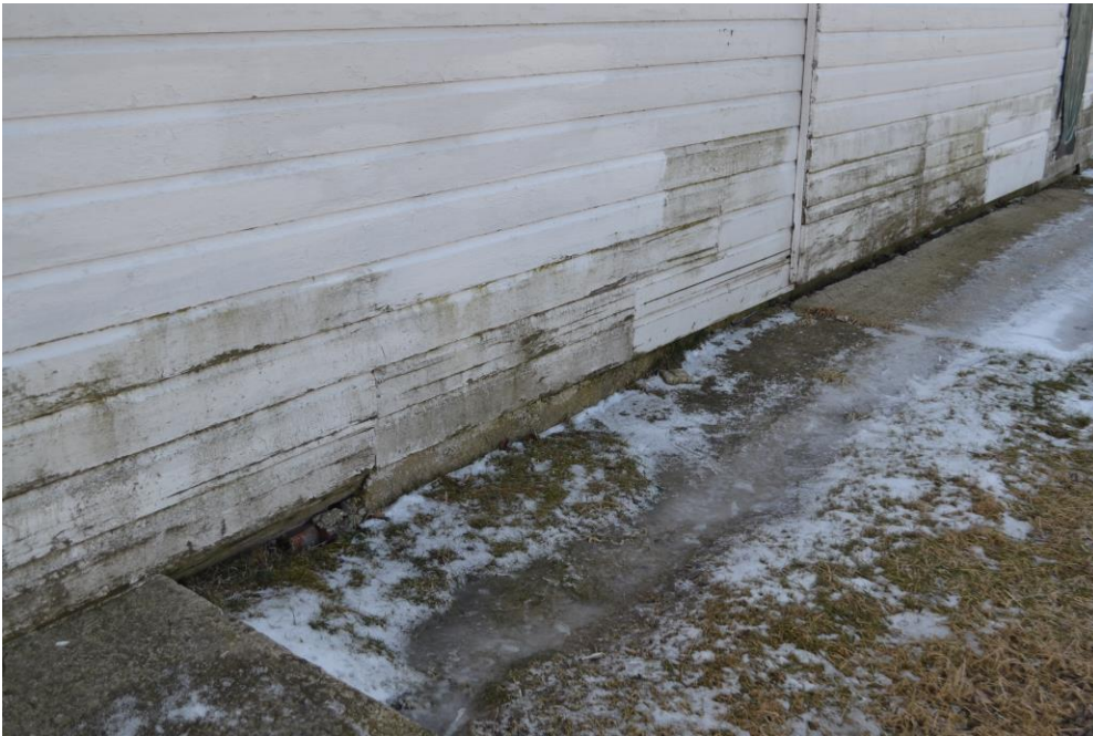
10. Algae and dampness leads to paint failure and wood rot.
