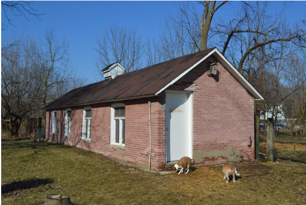
35-36. Chicken Coop. Above note inadequate mortar parging on front wall and settlement over modern metal entry door. Below note obvious settlement in mortar joints on back (north) wall.
