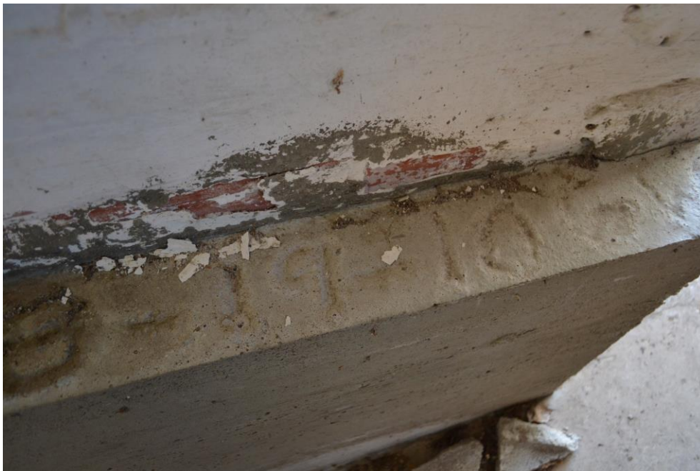
33-34. Dairy office in southwest corner features modest renovations and reinforcement, including masonry wall reinforcement along base of south basement masonry wall. Concrete buttresses were installed outside of the south wall sometime as an early reinforcement.
