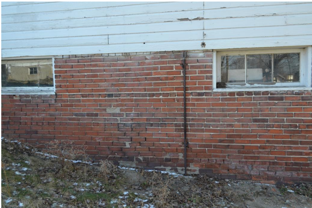
4. West basement wall demonstrates need for minor tuck-pointing near grade
