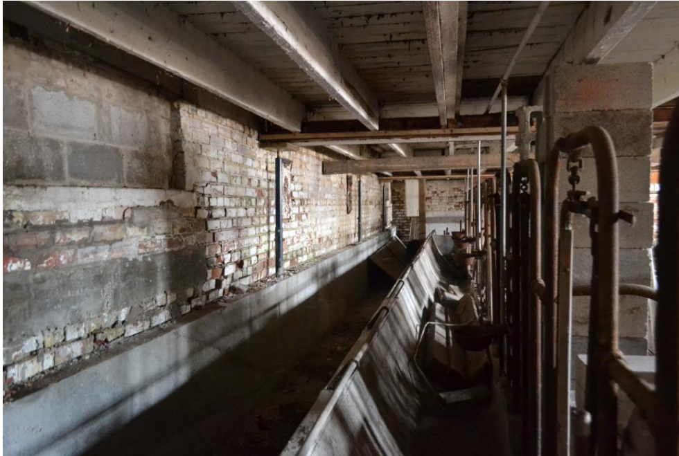
23-24. North basement wall shows signs of moisture settling down through the ground along the wall. Note that there were once windows in this wall, now blocked-in, which means that grade was likely raised a few feet at some time.
