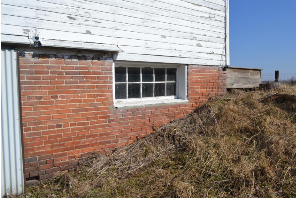
7. This best demonstrates the need for improved drainage and its lack creates need for masonry repair.
