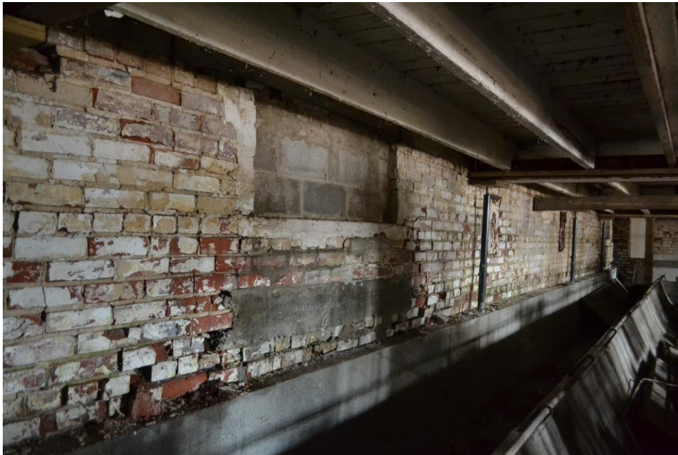
23-24. North basement wall shows signs of moisture settling down through the ground along the wall. Note that there were once windows in this wall, now blocked-in, which means that grade was likely raised a few feet at some time.
