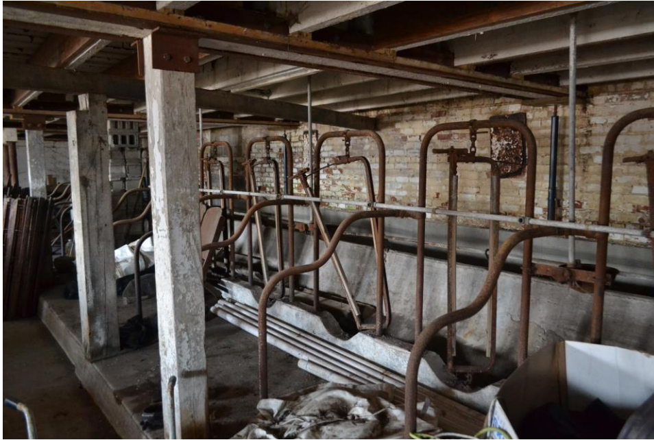
21-22. Example of extant cattle stanchions, drink bowls, and concrete troughs. Note post and beam reinforcement with steel angles (above and below).
