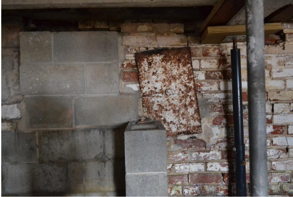
27-28. Some ad-hoc reinforcement of main level floor joists with concrete block and adjustable pipe columns. A traditional wood post and beam support could be exchanged with the ad-hoc materials.
