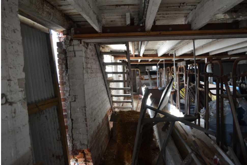
29. Looking west along south basement wall (above). Note separation of face brick on outside of wall and deterioration of masonry wall at base. 30. Passageway from milking floor to calving stall area (below).
