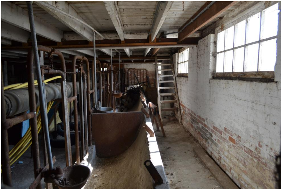
21-22. Example of extant cattle stanchions, drink bowls, and concrete troughs. Note post and beam reinforcement with steel angles (above and below).
