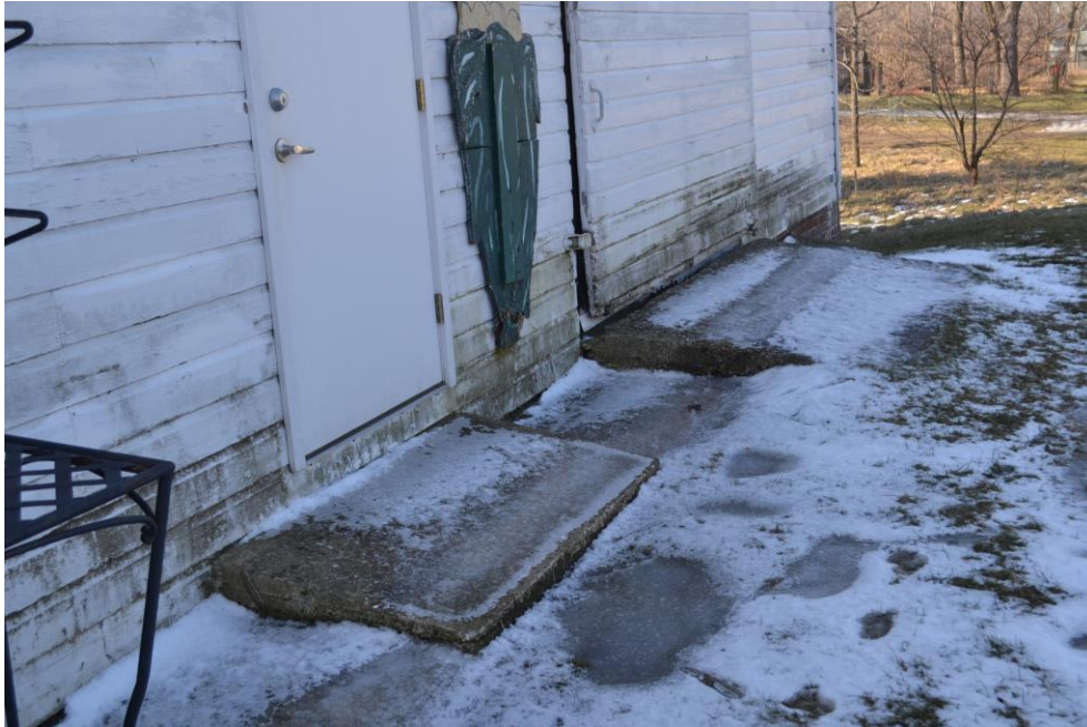
11. Rainwater is trapped along swale from concrete steps/pads into the building.
