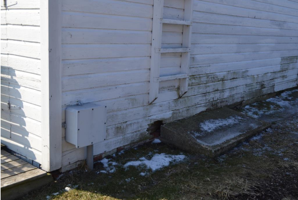
9. North wall suffers most from inadequate drainage because of water splash and lack of sun.
