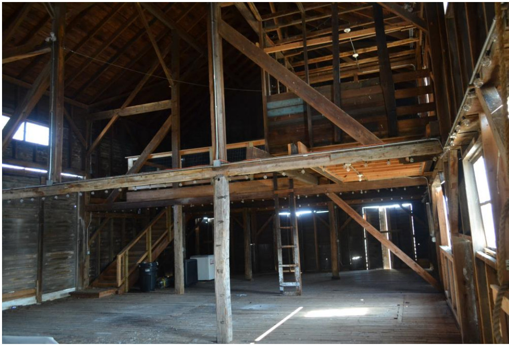
15. Looking east (top) and 16 west (bottom). Missing structural post in bottom photograph.
